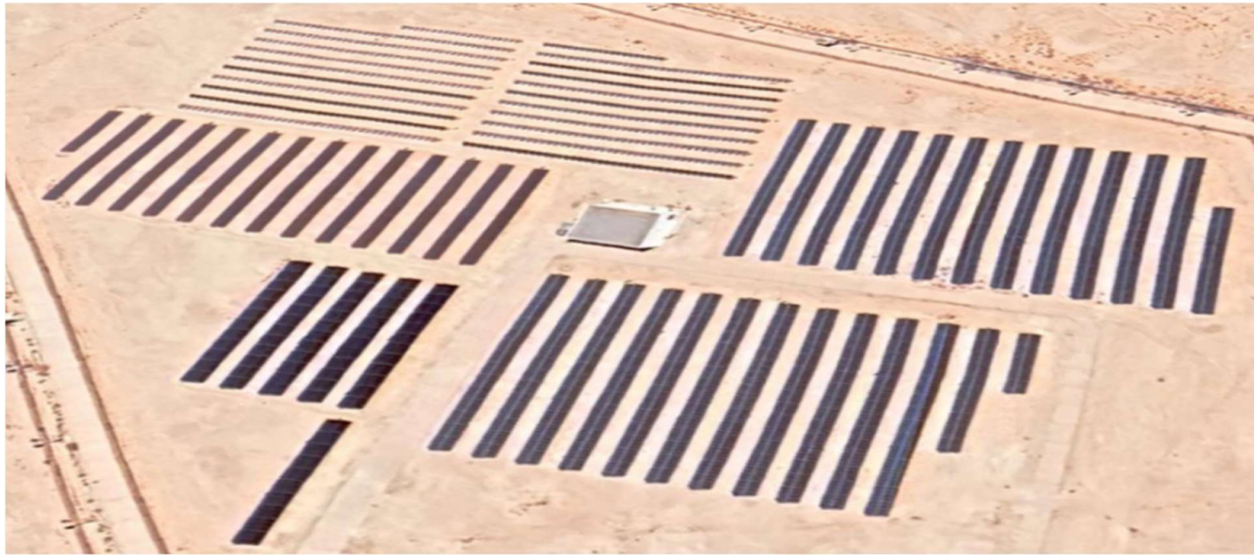
Figure 4: Ghardaïa Solar PV plant [38]
