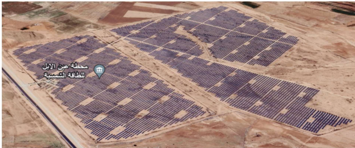
Figure 3: Djelfa solar PV plant [38]
